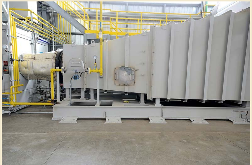
New co-generating Power Plant at Victoria Hospital Campus
