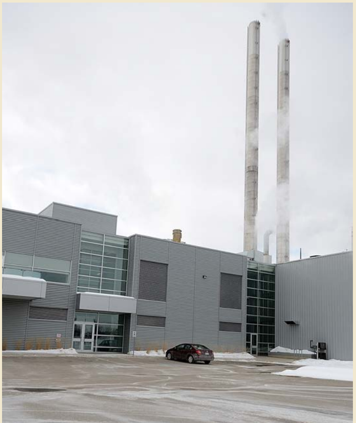
Power Plant at Victoria Hospital campus
