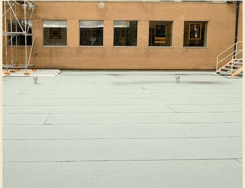
Newly completed roof replacement at VH
