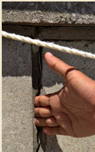
Deteriorated caulking
