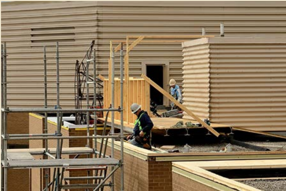
Working on the roof replacements
